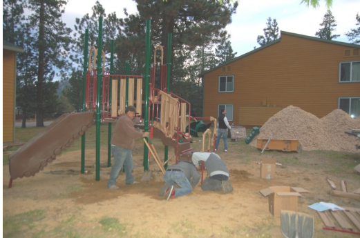
New Children's Play Equipment Under Construction at Sierra Garden Apartments
